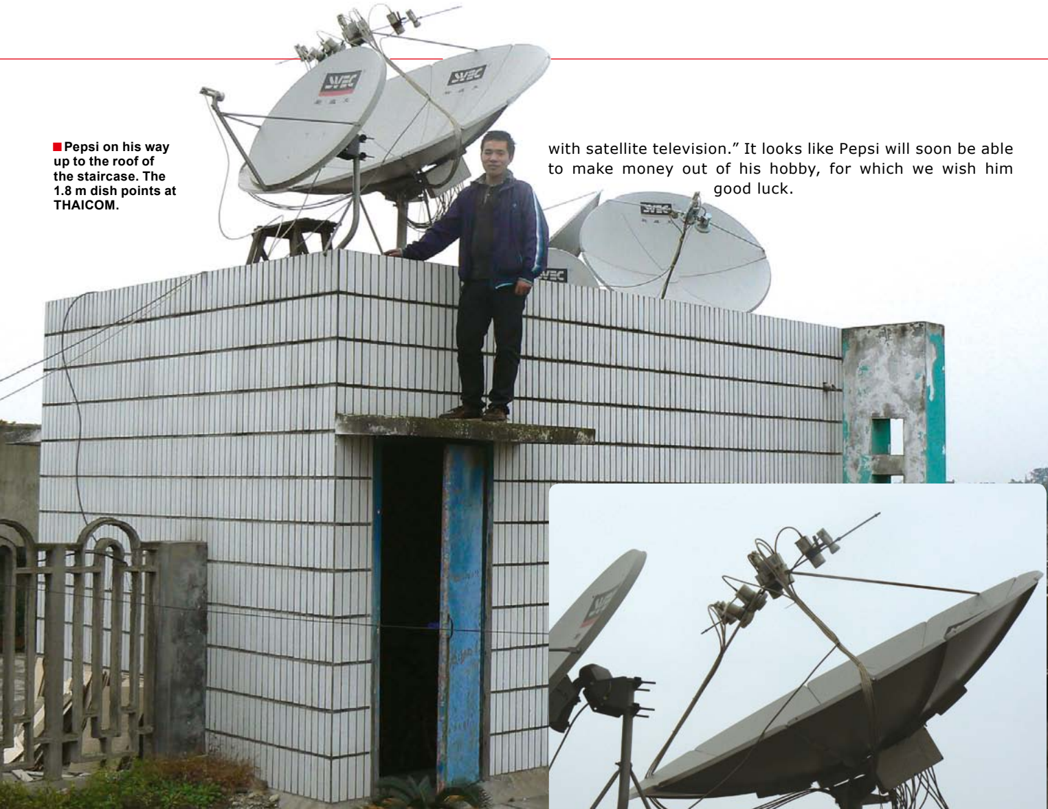
■ Using an extension rail Pepsi has converted his 2.4 m antenna into a multi-feed dish for reception of nine different satellites.
